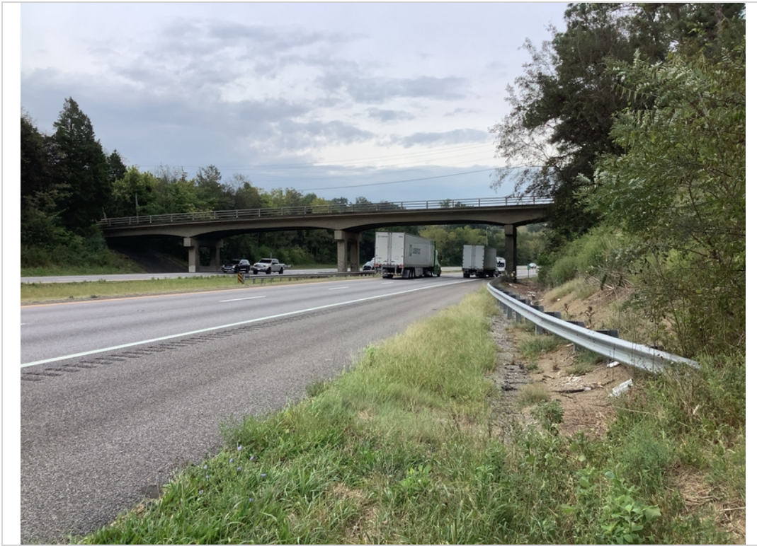
I-75 SB - Underpass back and elevation left
