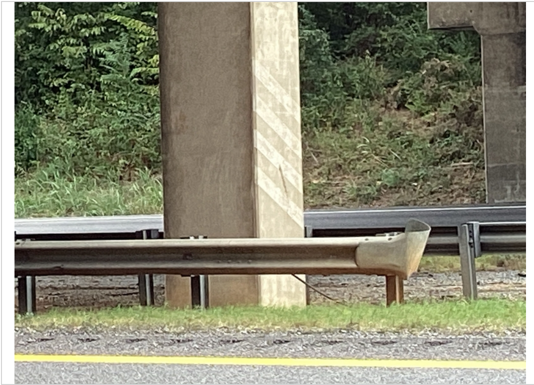
Column B right bent 2 - Popout
