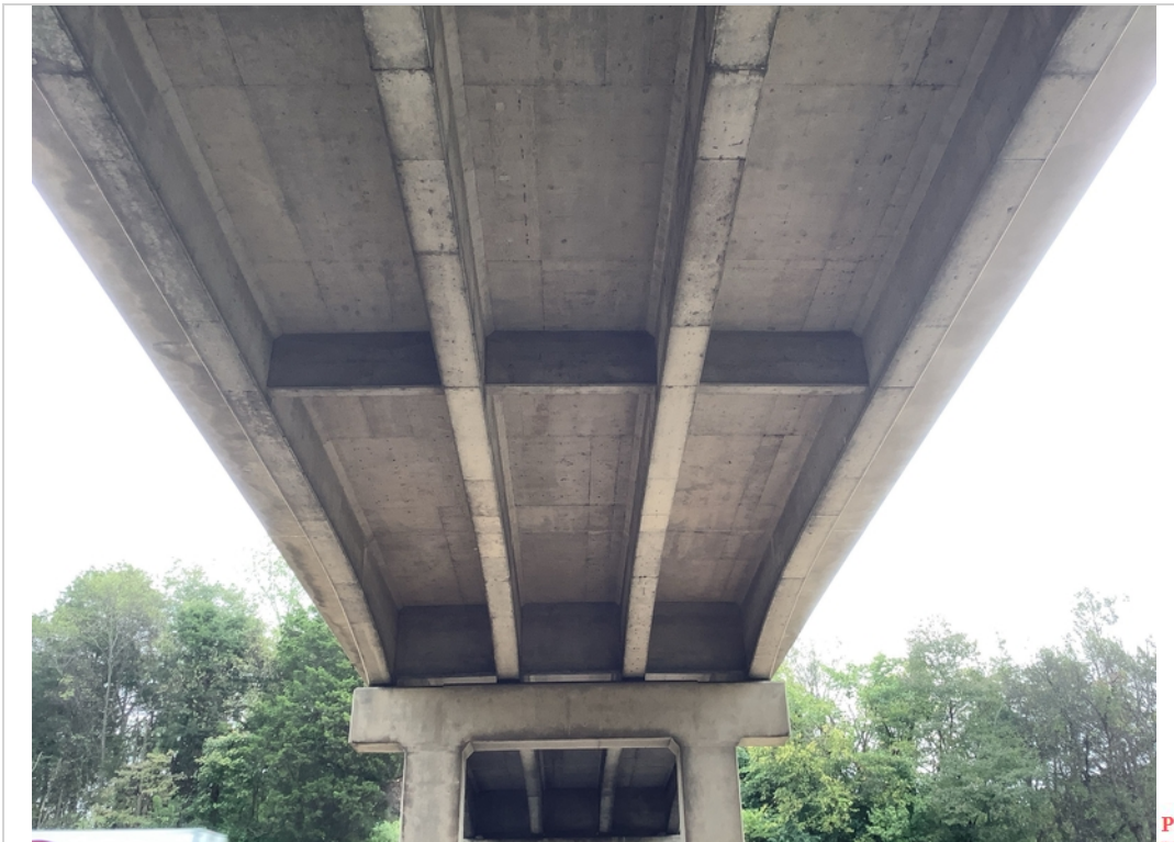
From bent 1 - View underneath
