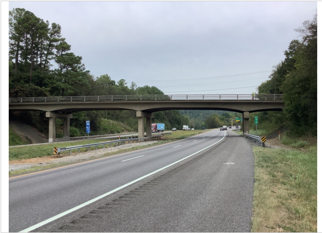
I-75 NB - Underpass forward
